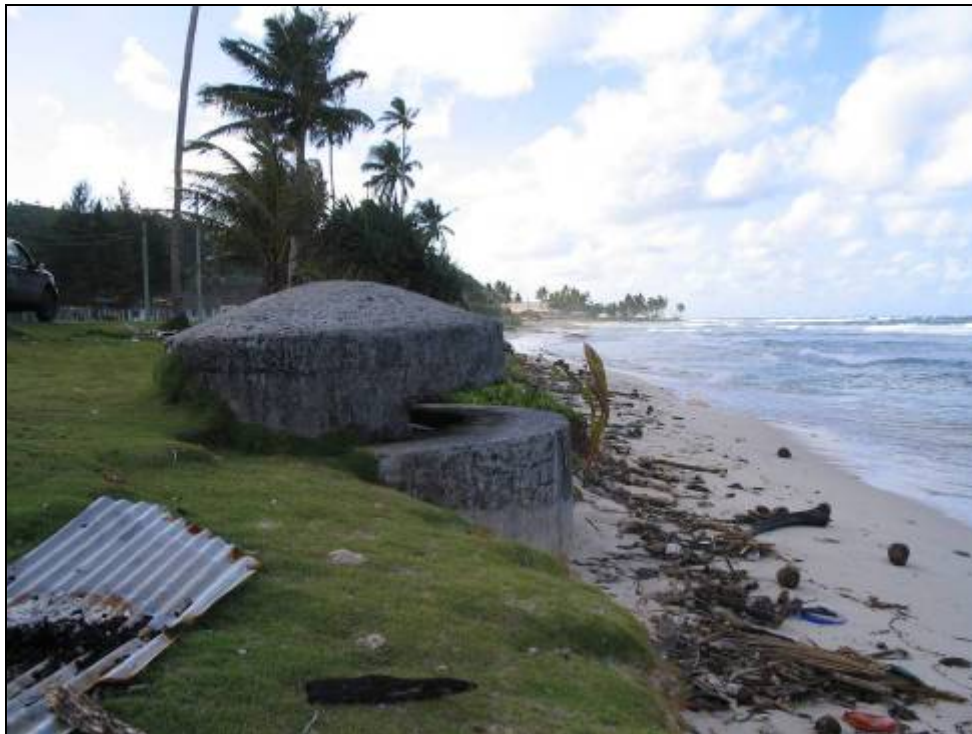
An empty World War II pillbox still stands guard on the beach near Alao. (NOAA ONMS)
